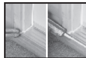
Figures 12 and 13: Caulk the sill crown and the front of the sill.
