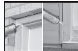
Figures 14 and 15: Caulk the jambs and the exterior trim.
